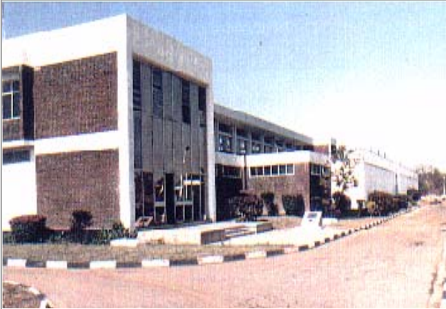
Lolanda water works, Kafue, Zambia
