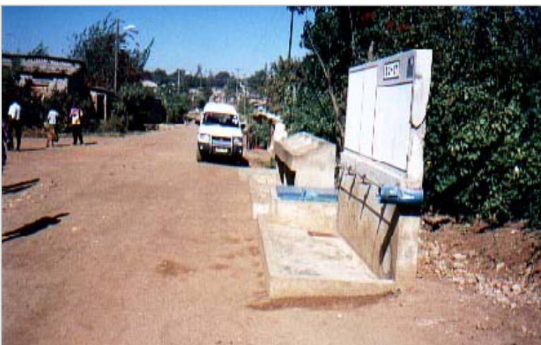
Some of the facilities provided at the GCWSS
